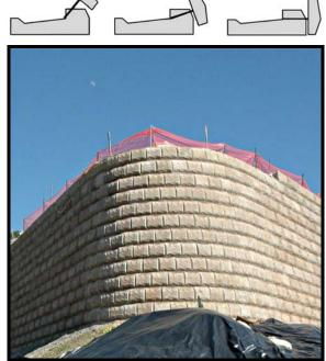
Outside corners are made using the LOCK+LOAD corner panels. When possible begin walls at outside corners to minimize panel trimming if "on bond" erection is required.
