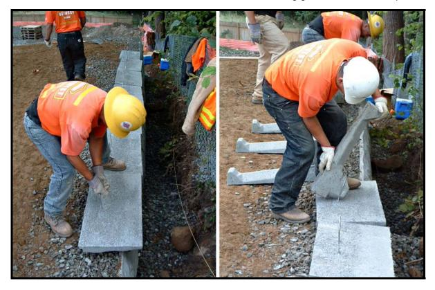
Use wedges between the counterfort head and the panel back to remove play and make the module rigid.
