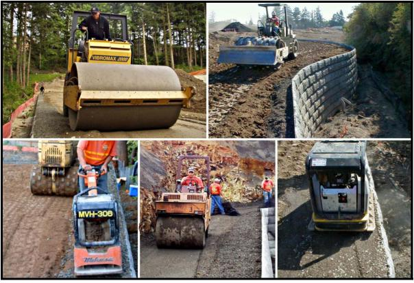
Even better compaction equipment are large the facings attachment to the soil mass. reversible diesel plate compactors with operating weights of 900 to 1100 lbs. [Examples: Wacker models (BPU-3345) or Multi Quip (MVH-200DA) or equivalent]. Roller compactors can safely be used to within 16" of the wall face. All compaction activity always begins with compacting over the tail of the counterfort first "locking" it into place.
