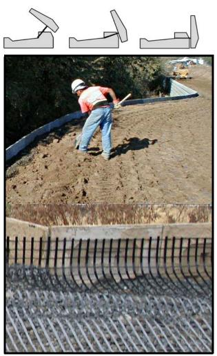
Now carefully backfill over the grid, to the top of wall panel, keeping the geo-grid tight and free of wrinkles., A minimum of 2 foot of select material is to be maintained at the wall face. Compact as previously described beginning over the tail of the counterfort to the panel back and then toward the back end of the geo-grid Insure that the geogrid remains in contact with the panel back after compaction.
